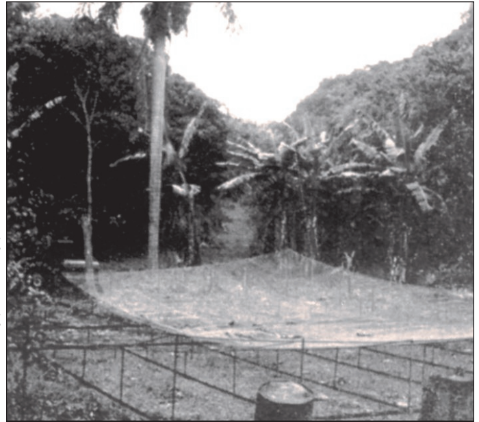
In 1968 W1FZJ/KP4 made a 50' [15.2 m] square dish for 432 EME tests. The dish was later planned to be expanded to 150' for use on 144. A movable feed was to be mounted atop a 60' tower in the center of the dish. Unfortunately, Sam never finished the bigger version due to his illness and passing.
